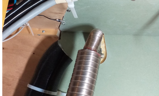
Sensor above black pipe Black pipe: Intake heater Shiny tubing: Exhaust (Note that the exhaust should be gas tight)
