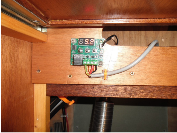
Sensor above black pipe Black pipe: Intake heater Shiny tubing: Exhaust (Note that the exhaust should be gas tight)
